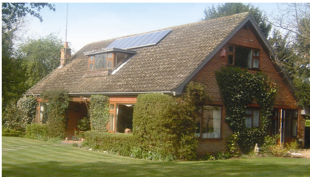
A typical 2kWp solar PV system on a detached house
